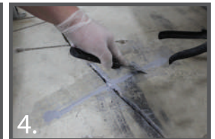
4. Scrape away excess epoxy
