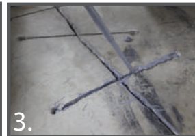
3. Apply epoxy over the Concrete Crack Lock®
