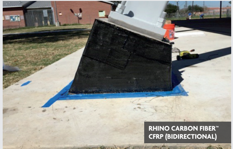
CRACKED THRUST BLOCK
