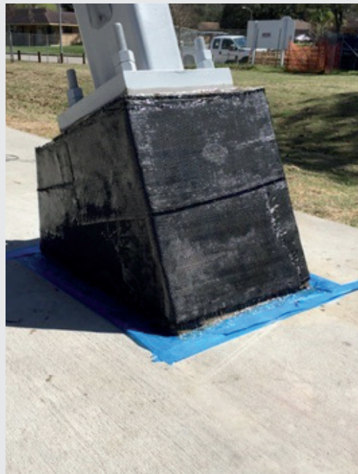
CRACKED THRUST BLOCK
