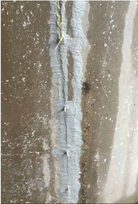
CRACK INJECTION
