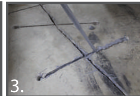
3. Apply epoxy over the Concrete Crack Lock®
