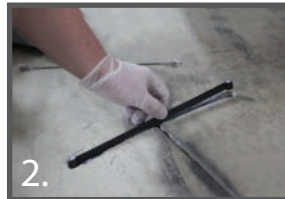
2. Press the Concrete Crack Lock® into epoxy
